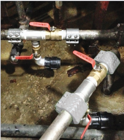
Completed repair of new PVC pipe for sewage disposal
