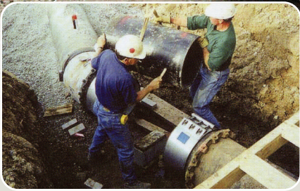
▲ Repair work for pipes replaced underground
