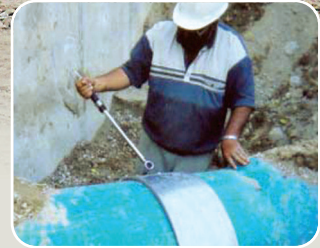
▲ UK: buried water supply pipes
