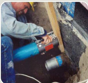
▲ U.S.: sewerage repair work
