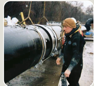
▲ UK: district heating work
