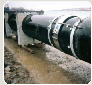
▲ U.S.: nuclear power plant
