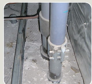
▲ PVC + Steel Pipe Connection
